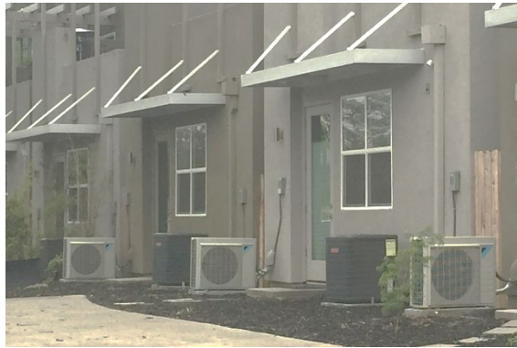
Figure 3-21 – Do not leave HVAC and other equipment unshielded
