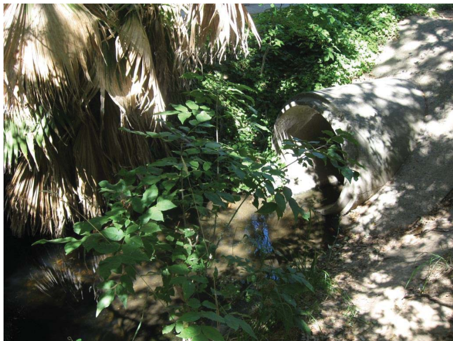
Photo 3-2. Drainage Channel Outlet to Arcade Creek – Near Sweet Gum Court
