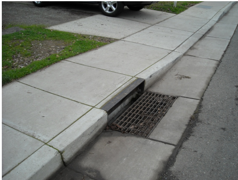
Photo 3-4. Curb, Gutter and Inlet – Mariposa Avenue at Cina Way
