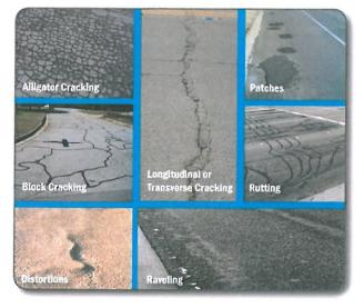
quality, rutting), GPS, and surface distress data is collected continuously and seamlessly by our pavement technician team using our automated data collection vehicle which makes available a wide range of survey technologies. Our pavement distress data collection process involves the use of customized, integrated keyboards, and laser scanning which are all used to collect the type, severity, extent, start and stop points of all the StreetSaver® pavement surface distresses.
